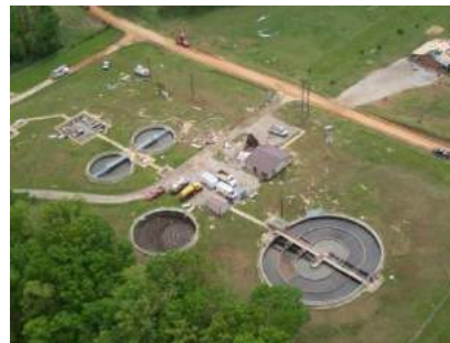
Figure 5: Wastewater treatment plant at Willow Springs. Photo/KY3 Springfield News
